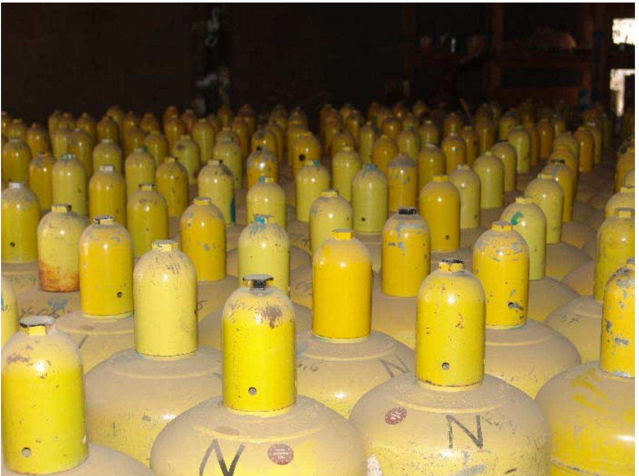
Picture 1. Chlorine tanks at the Sana'a water treatment plan. A simulation exercise was conducted at this facility as an input into the draft contingency plan.
