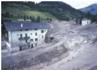
Flourite Dam Failure, Stava, Italy, 1995
