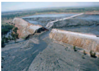
Dam Failure, Aznalcóllar, Spain, 1998
